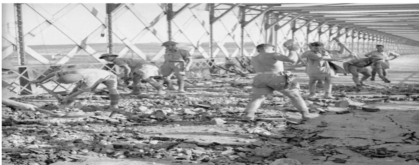
British engineers repair the damage to the Primosole bridge over the Simeto River after its capture in July 1943. Control of the Primosole and Malati bridges was essential to allow the British advance in the Catania plain and prevent their destruction by retreating Axis forces. Photo by Sergeant Gladstone, No. 2 Army Film & Photographic Unit. Imperial War Museums.
